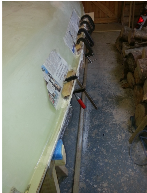
Figure 16: Again with protection using masking tape and newspaper, the strips are clamped in with epoxy and filler. Cling-film is used to make sure that the wooden clamping blocks don't end up being incorporated into it
