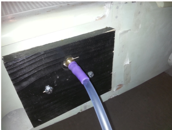
Figure 6: Makeshift blanking plate covering a transom hatch
