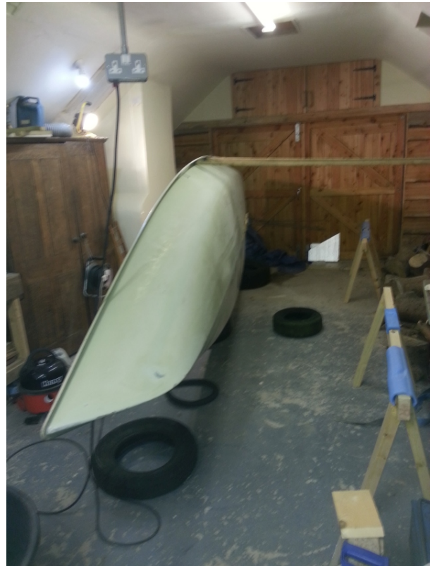
Figure 11: Hull propped on its side making the defect easy to prepare and fill
